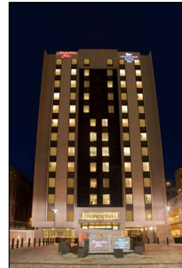
Renovated View of Façade →
